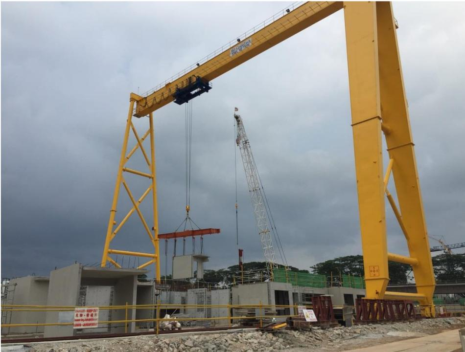
*Figure 3: Johnny championed the use of PPVC - Prefabricated, Prefinished Volumetric Construction, a new technology that improved site productivity and safety.*
